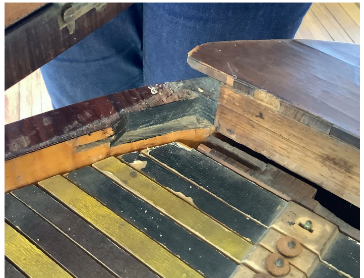
Figure 3. Recess cut into the treble-most bentside curve, perhaps to free the corner of a missing horizontal panel that would have fit in neighboring slots. The key ends have been cut at an angle to fit the curve.
